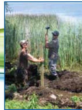
Installing wildlife barrier fencing along Causeway
