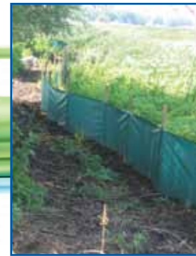
Installing wildlife barrier fencing along Causeway
